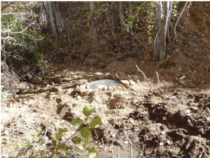
Huni Spring development 2013, showing spring box.
