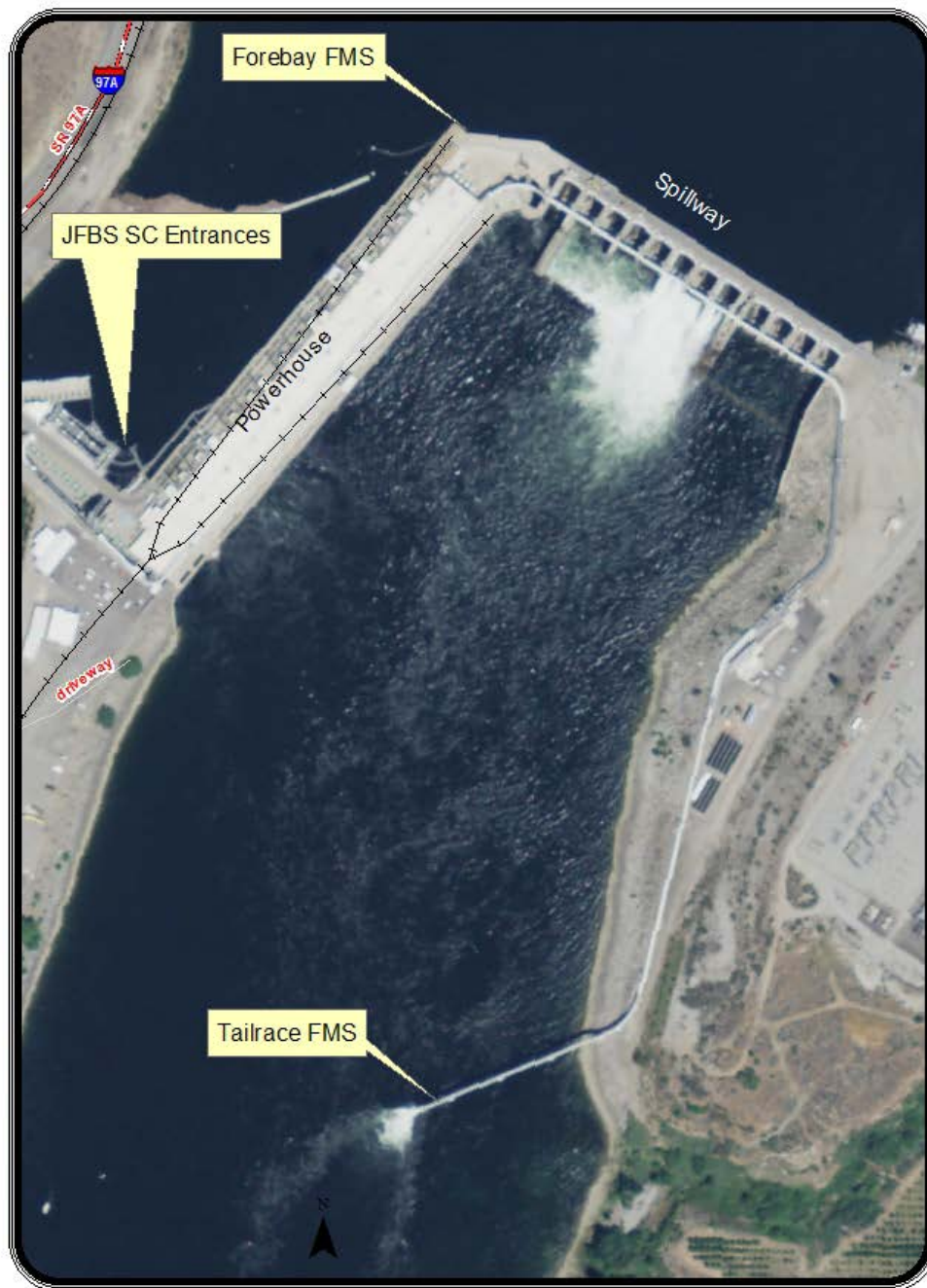
Figure 2-1. Location of the forebay and tailrace FMSs, and the JFBS SC entrances
