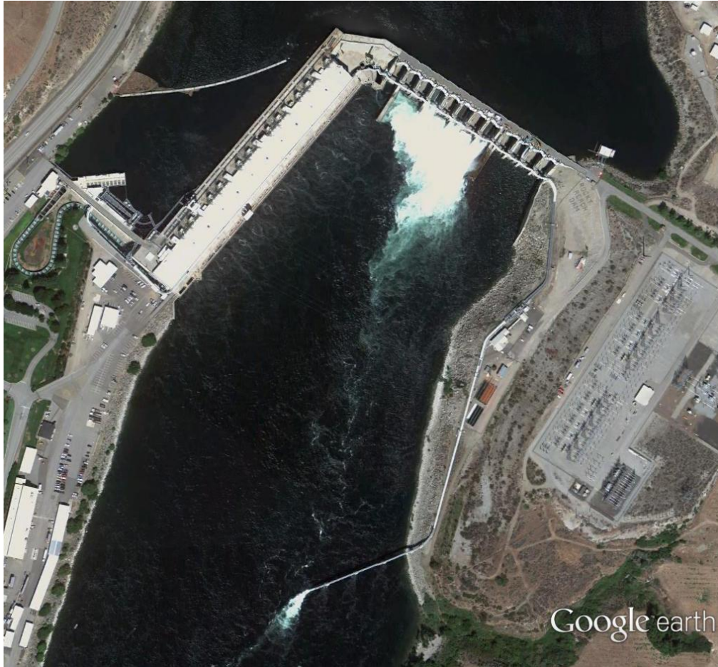
Figure 2. Aerial view of Rocky Reach Dam (Google Earth 2012).
