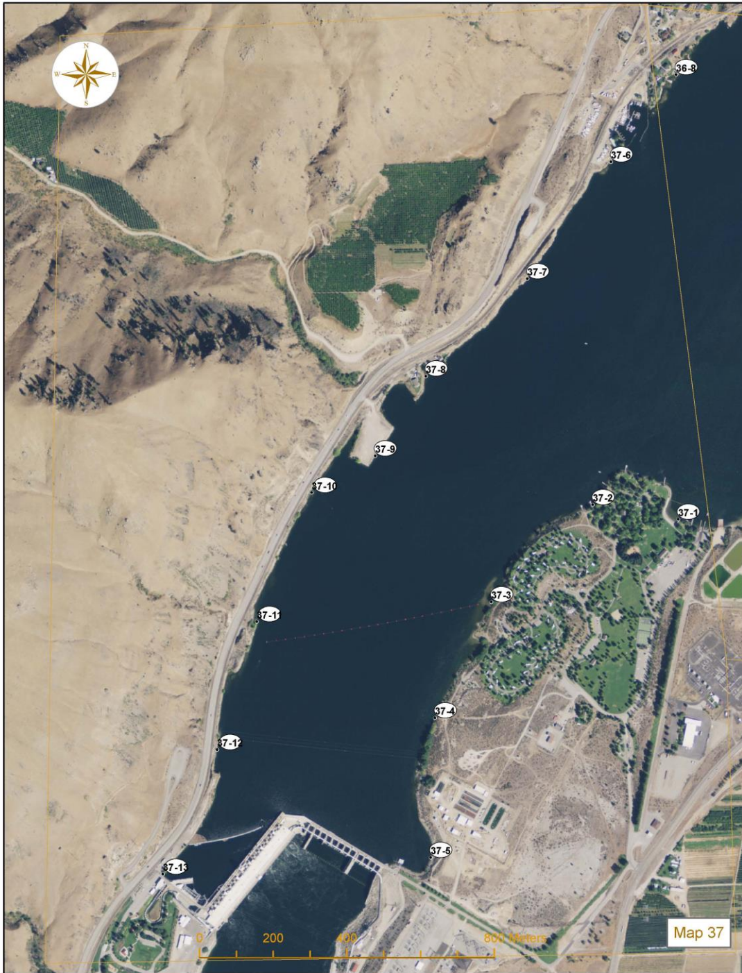
Figure 2. One of the 37 sections and associated sites including the Rocky Reach Hydroelectric Project.
