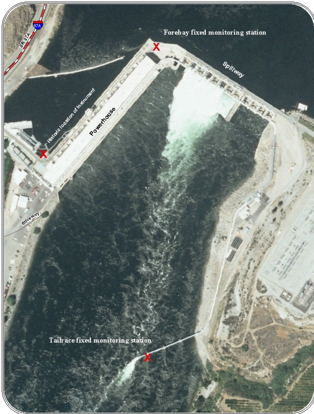
Figure 2. Location of forebay and tailrace fixed monitoring stations at Rocky Reach Project.
