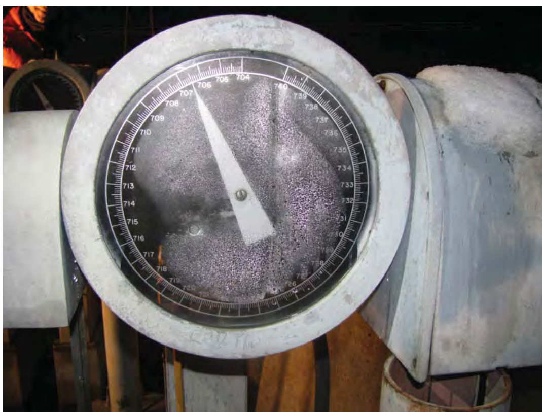
Photo 6: Tailwater gage used to record the tailwater level. The Collection Chamber gage is in the background to the left. The difference between these two readings indicates the head drop across the fishway entrance. (Photo by NHC)
