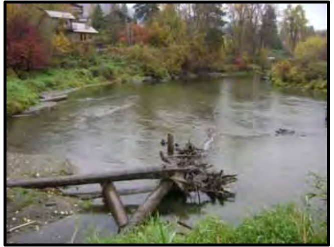
Outlet and Wenatchee side channel.
