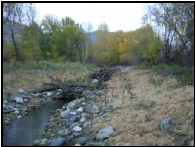
Looking down outlet channel (2).
