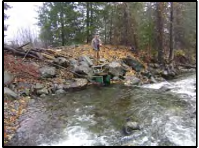
Diversion at Wolf Creek (2).
