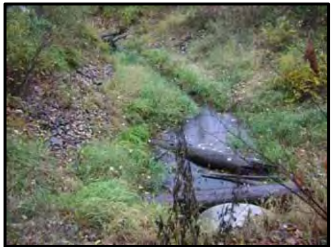
Channel leading to Blackbird Pond and culvert under trail.
