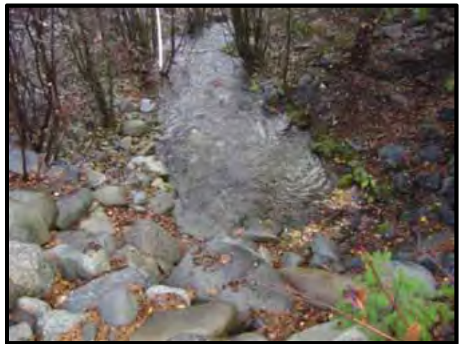
Diversion Channel above upper pond.
