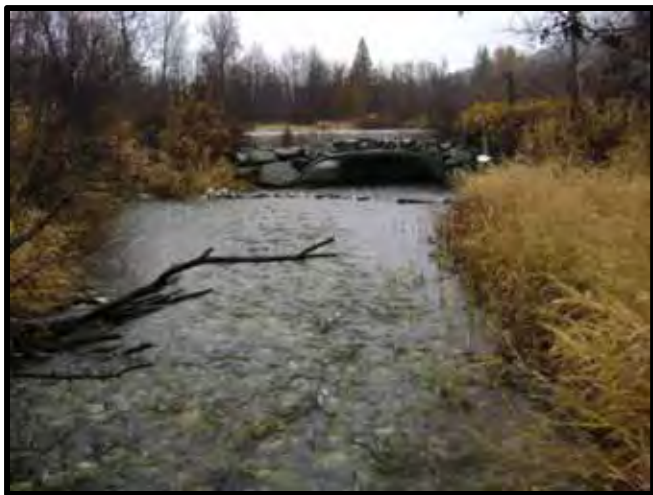
Culvert under Wolf Creek Road.
