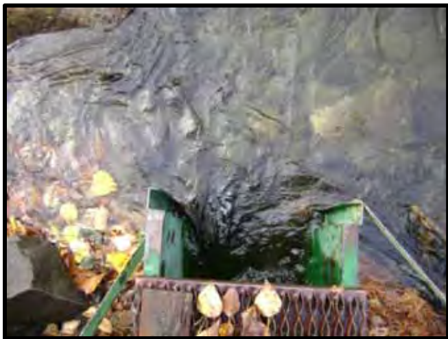
Diversion at Wolf Creek (3).
