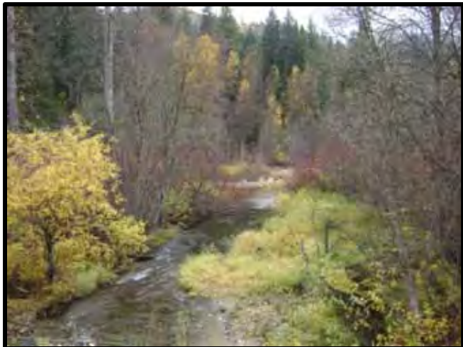
Outlet downstream of culvert.
