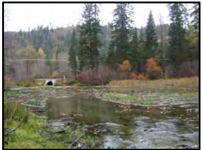
Looking back at inlet culvert.
