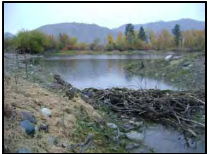
Looking up at outlet.
