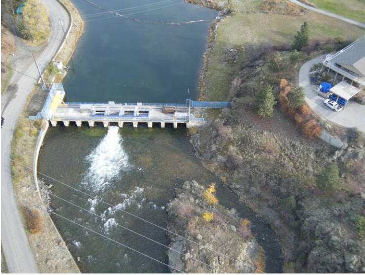
Skaha Lake Outlet Dam
