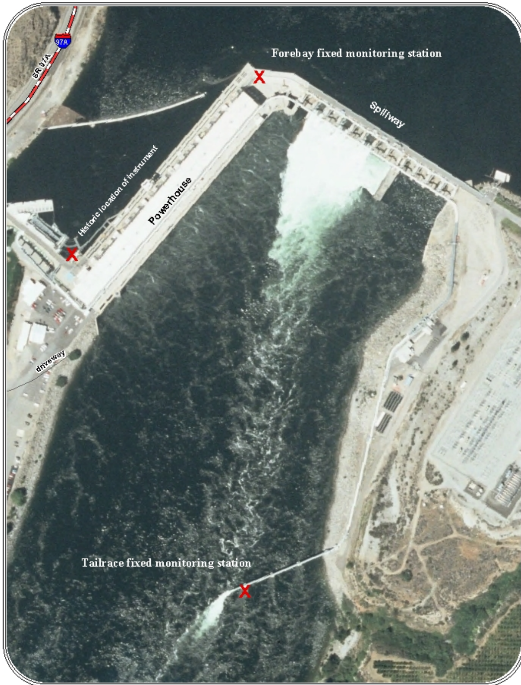
Figure 2. Location of forebay and tailrace fixed monitoring stations at Rocky Reach Project.
