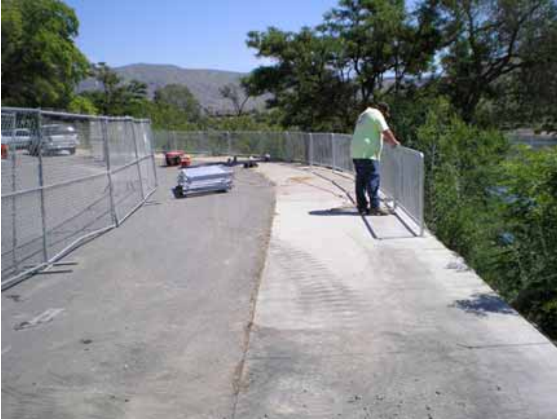
New handrail installation in progress [June 2007].
