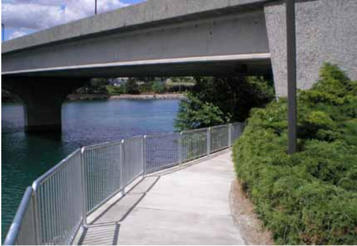
Finished sidewalk and handrail placement [June 2007].
