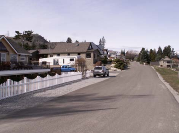
From the intersection of Terrace Avenue and Water St. looking west. Typical homes.
