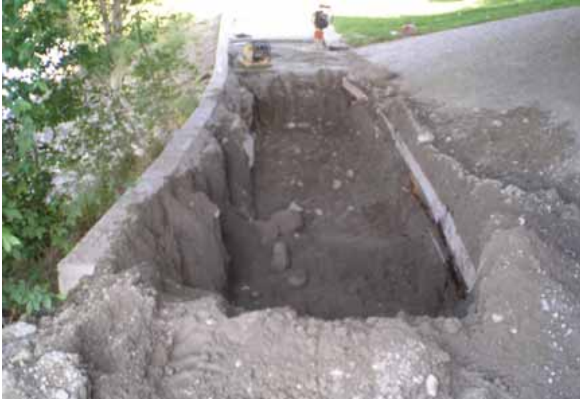
The voided area and ultimate limits of the repair [June 2007].
