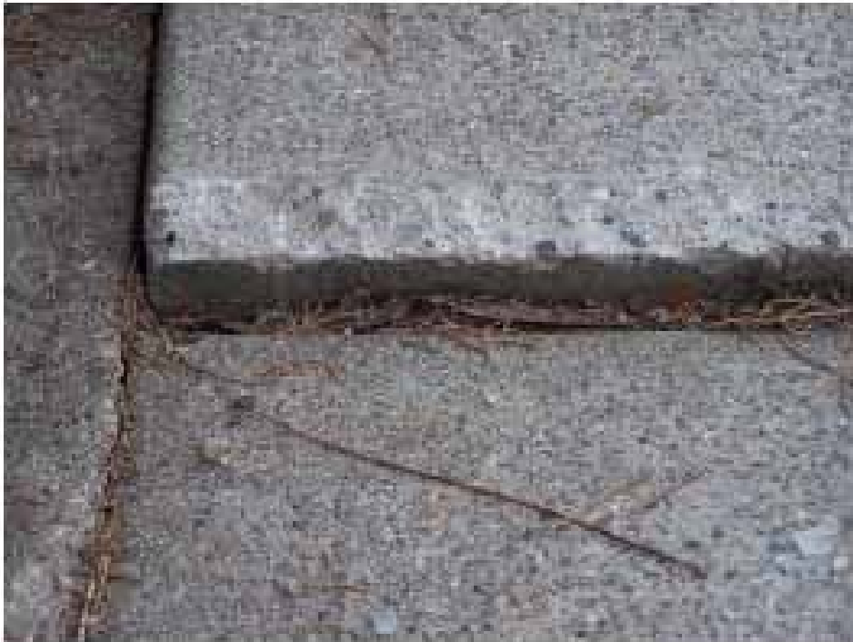
Sidewalk prior to repair [June 2007].
