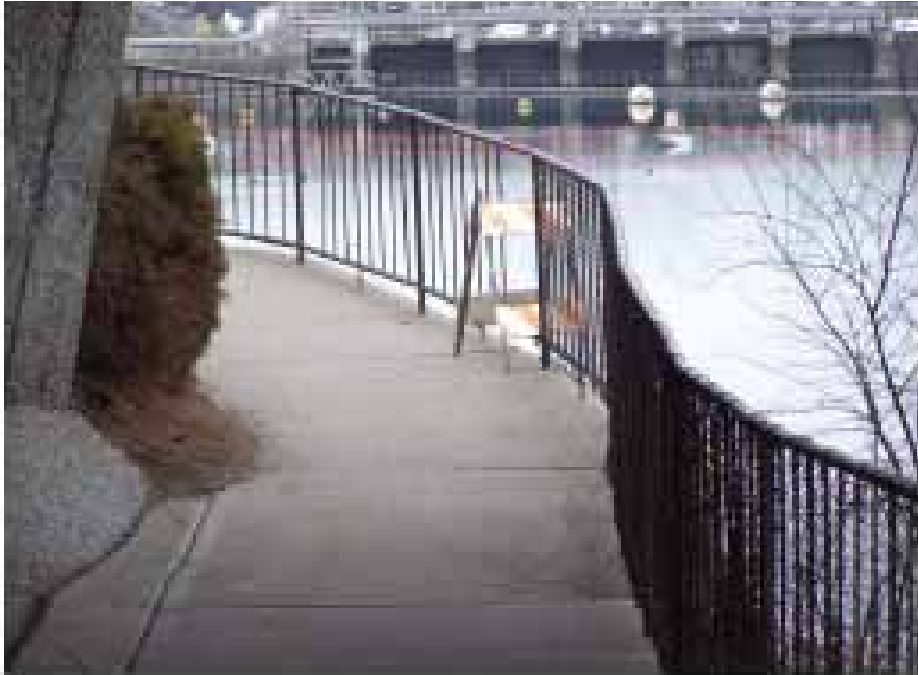
Damaged handrail [June 2007].
