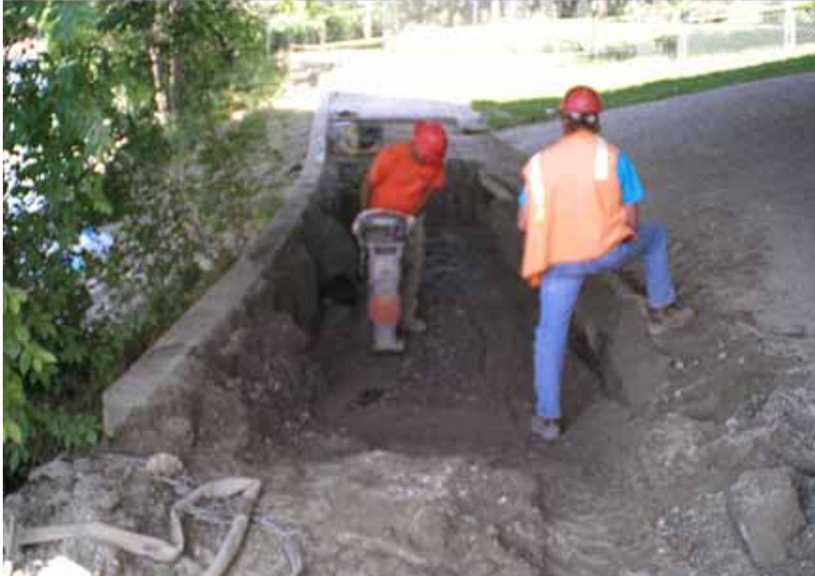
Sidewalk subgrade placement [June 2007].
