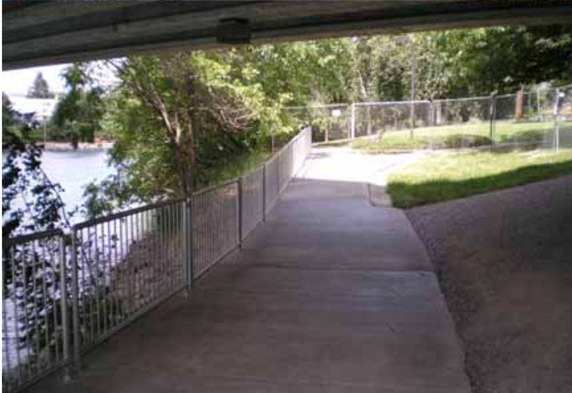
Finished sidewalk and handrail placement [June 2007].
