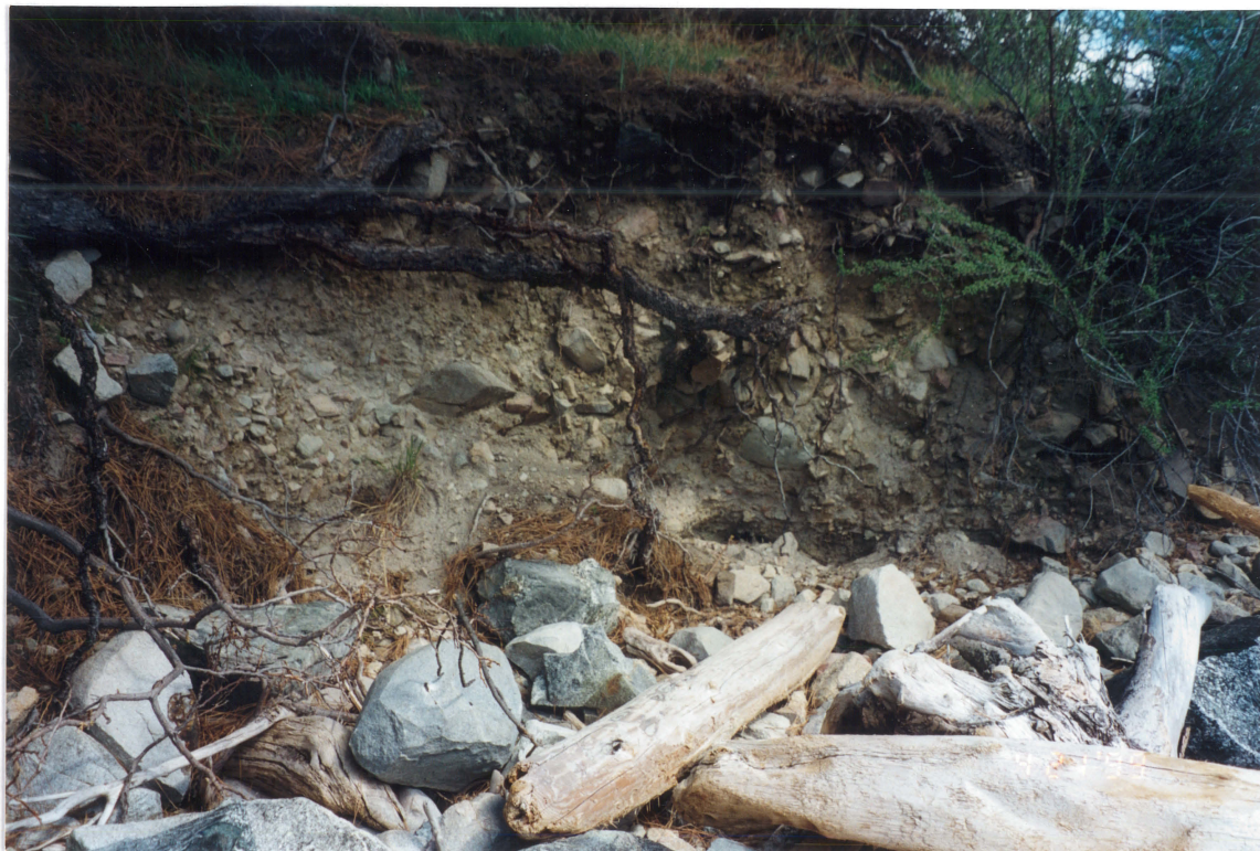
Exposed tree root close-up of area A1
