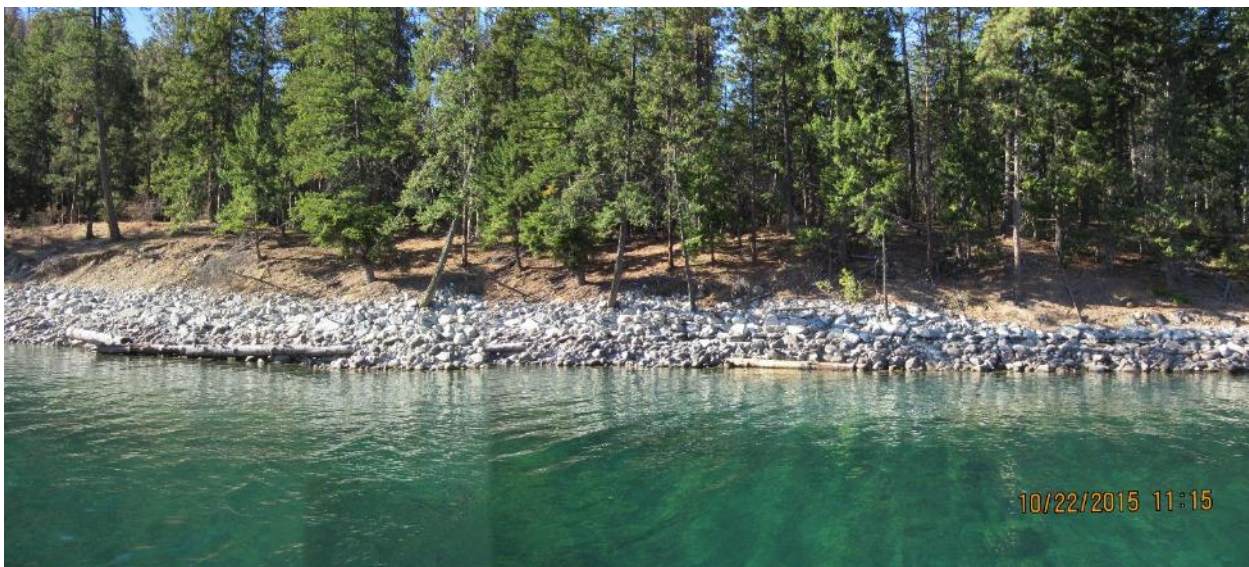
Refrigerator Harbor Treatment Zone C, D and E
