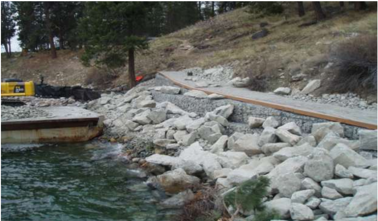
Prince Creek work in progress showing treatment area B with fabric cloth and side/surface view of gabion access path.
