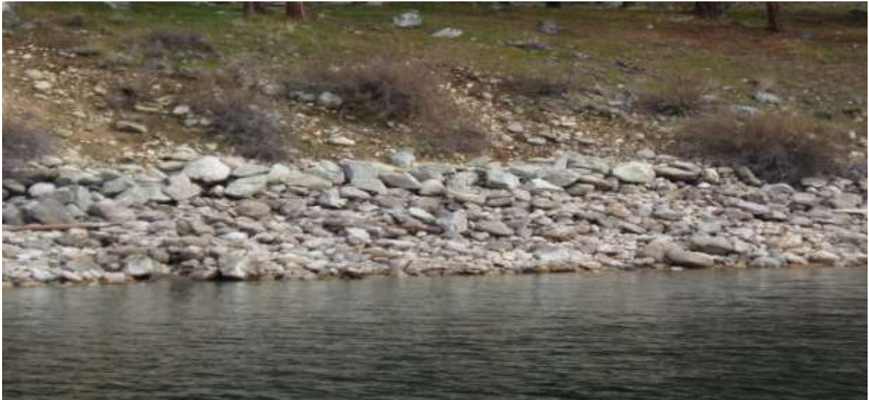
Treatment zone A ~ 20 feet Single/Double rock treatment.
