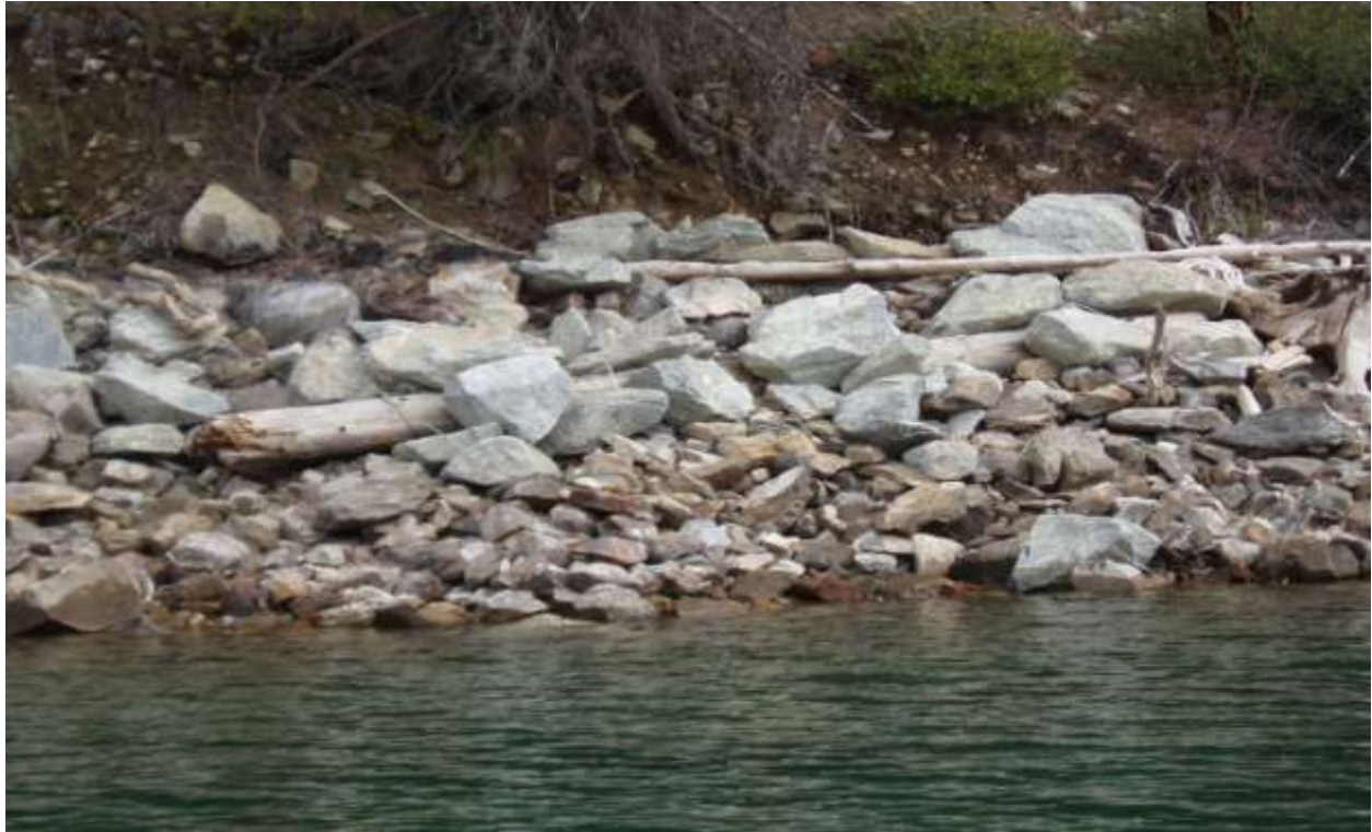
Prince Creek D4 treatment with LWD #11 Placed, triple cabled and rocked.
