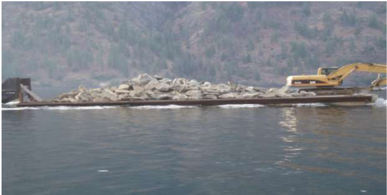
Courtney Tug and Barge provided 5 loads of rock and equipment to the sites.
