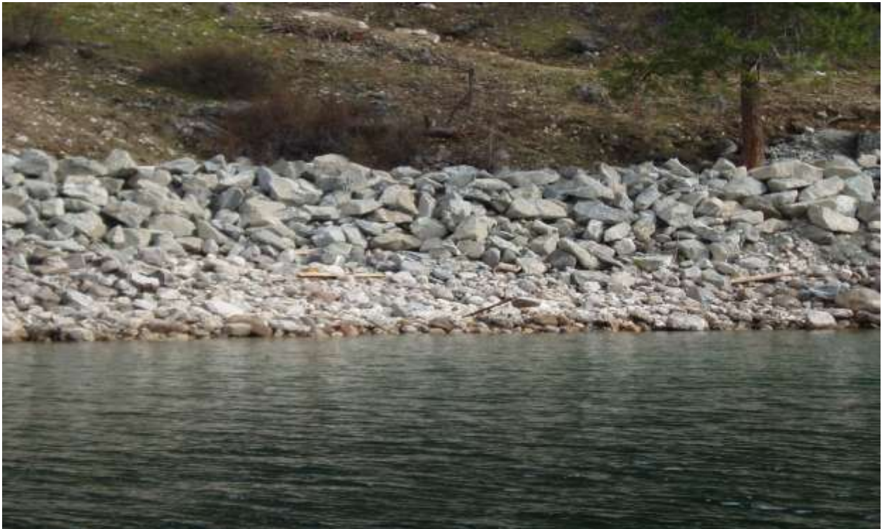
Treatment zone B ~90 feet old wood crib wall, no excavation just fabric cloth and protection of vertical crib wall with large rock amouring.
