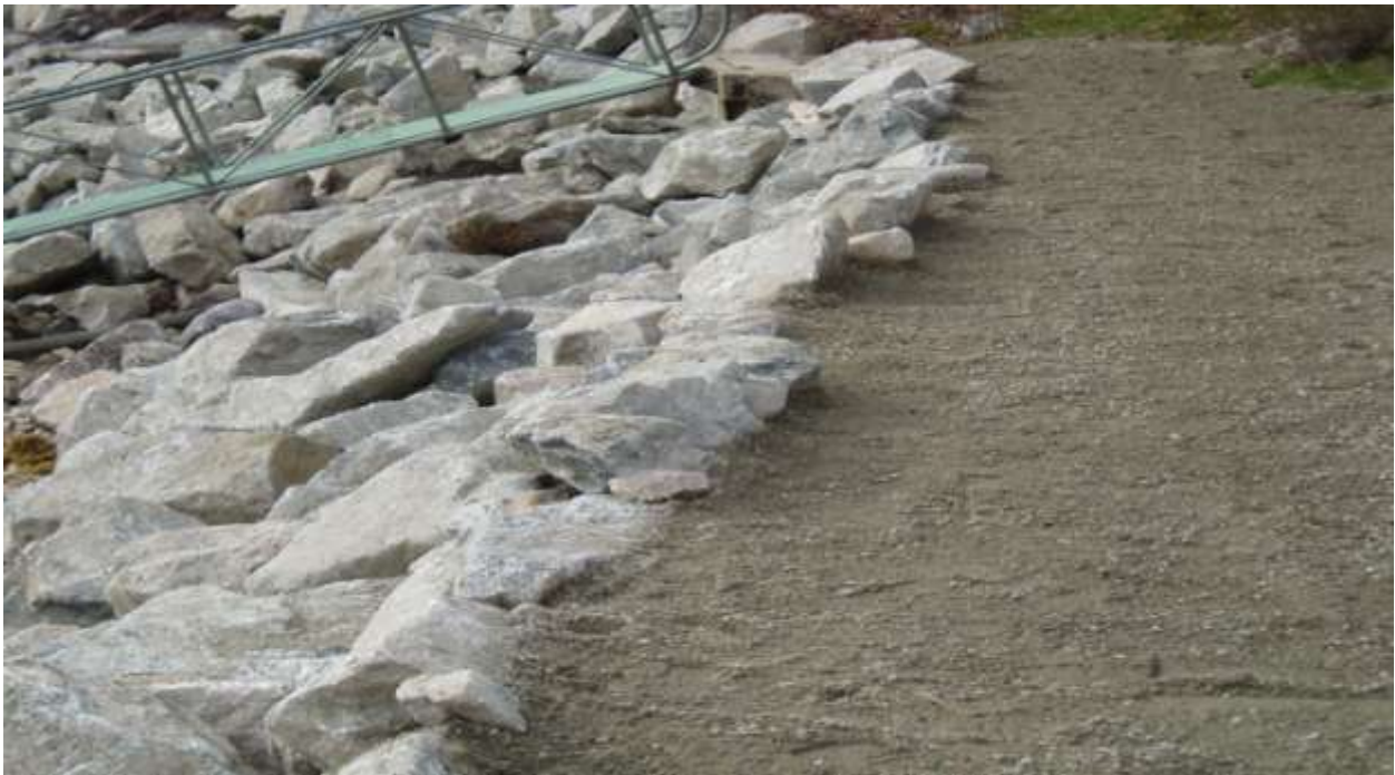
Side and top view of C2 gravel top, (Note slope profile better than 1/1)
