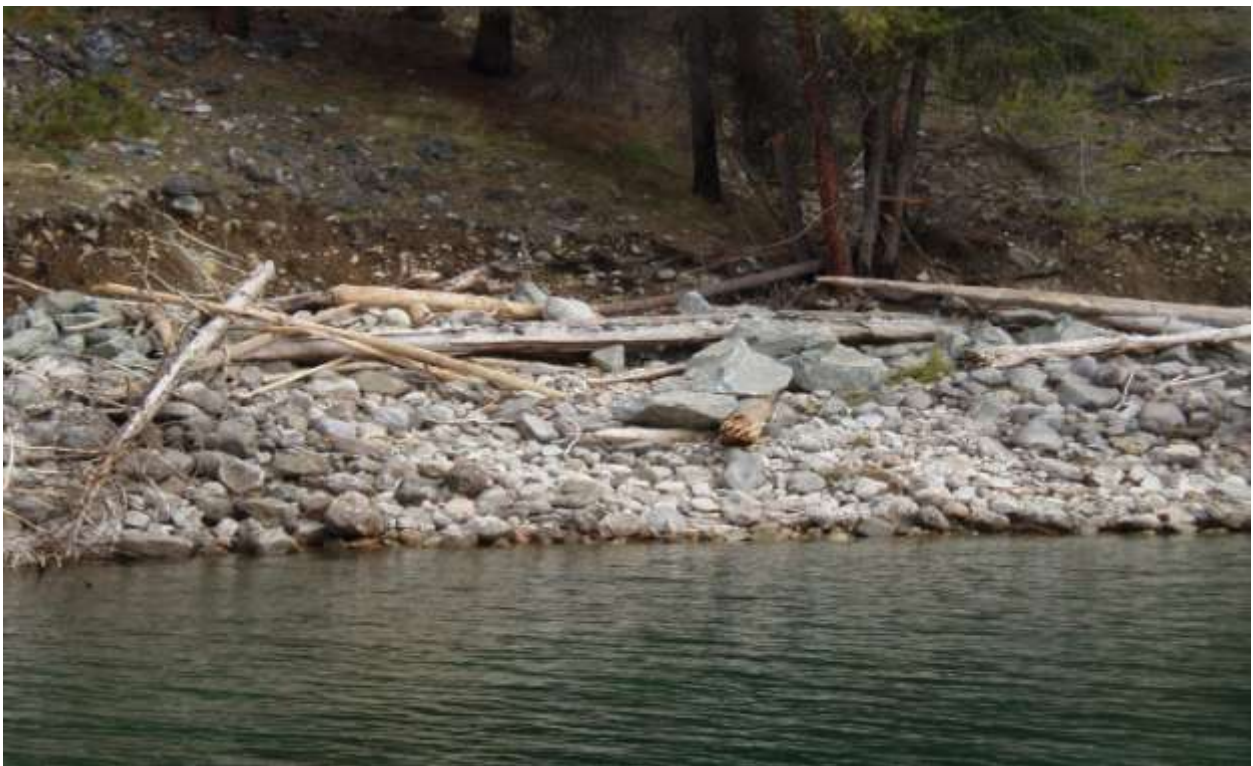
Prince Creek treatment E1 middle LWD #3 Natural top rocked, LWD #5 placed with triple cables and rocked.
