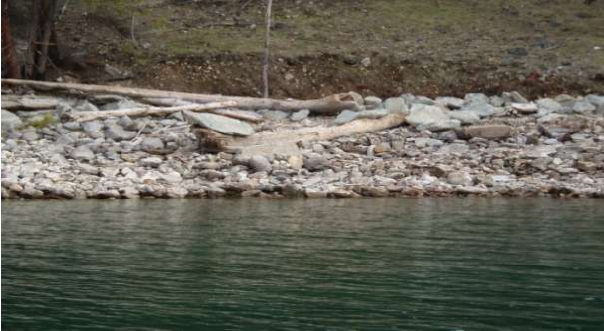
Prince Creek E1 treatment LWD #6 Placed, triple cable and rocked, double rocked shoreline with native wood moved behind rocks.
