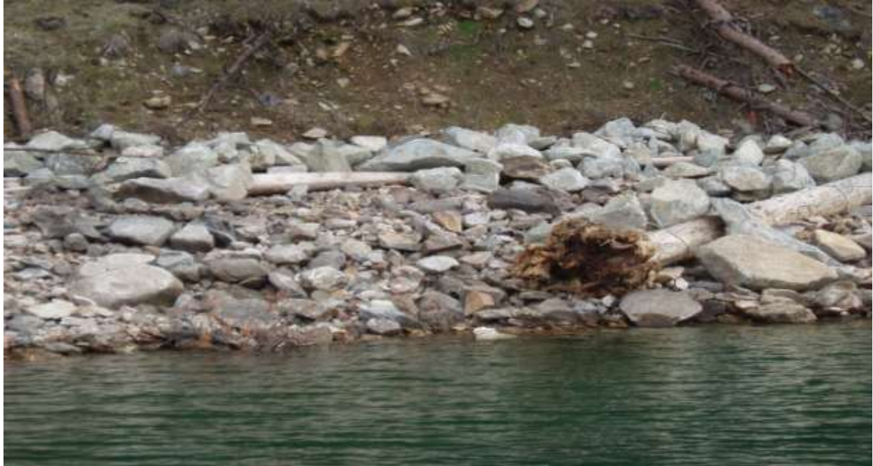
Prince Creek treatment E4~ 70 feet, with LWD # 4 Natural rocked (top left) and LWD #10 Placed, triple cabled and rocked (lower right).
