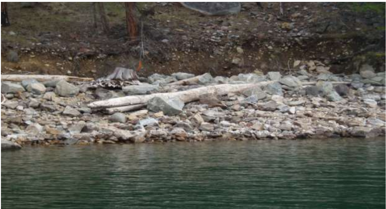
Prince Creek E2 double rock treatment with LWD # 7 placed triple cabled and rocked.
