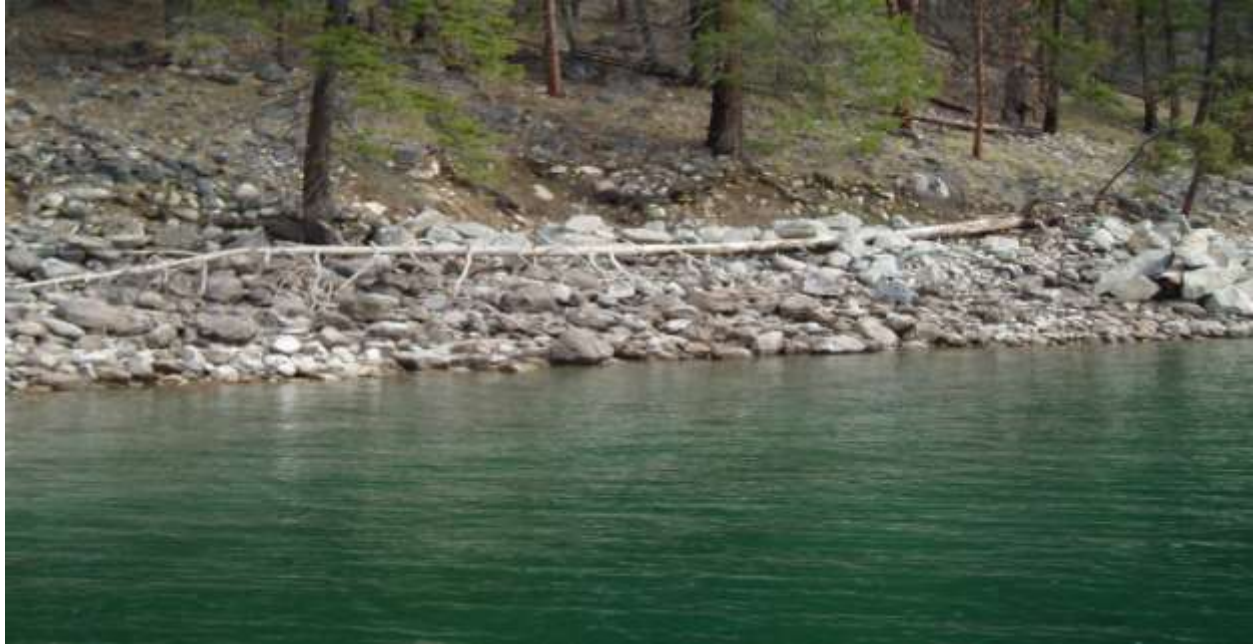
Treatment zone D2/D3 ~40 feet single/double rock with LWD #1 Natural rock anchored.
