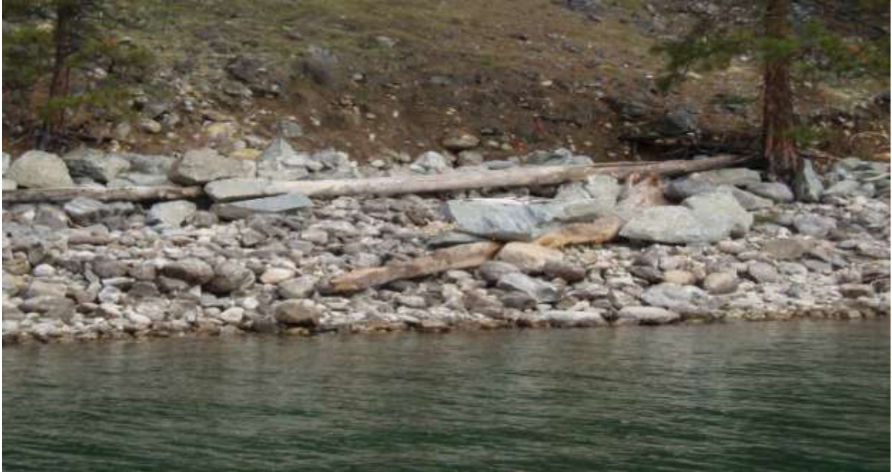
Treatment E1 Double rocked with LWD #2 Natural upper portion, lower LWD # 4 Placed cabled and rocked.
