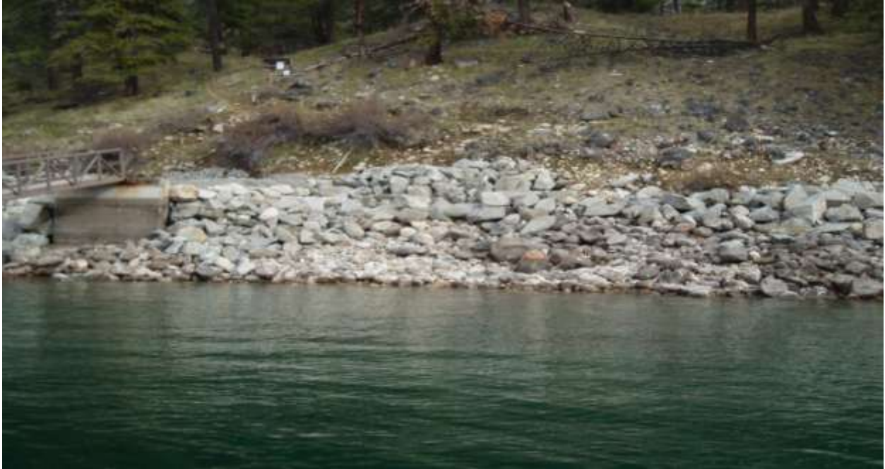
Treatment zone C2 ~ 35 feet of T1 treatment
