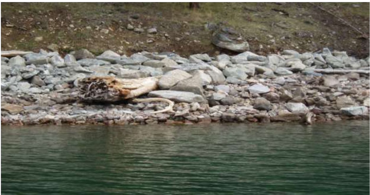
Prince Creek E3-E4 treatment LWD # 9 Placed, triple cabled and rockered.
