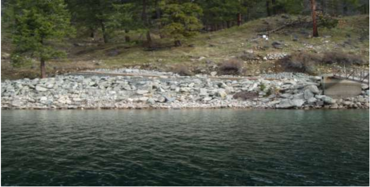
Treatment zone C1 ~90 feet recreational access trail on gabion wall, toe excavation occurred in this treatment to stabilize gabion basket placement.
