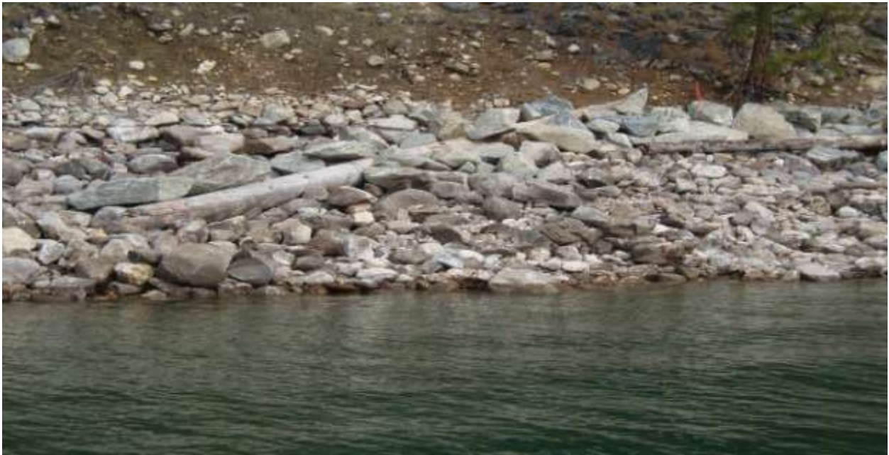
Treatment E1 beginning ~120 feet LWD #3 Placed double cabled and rocked, with LWD #2 Natural upper left rocked
