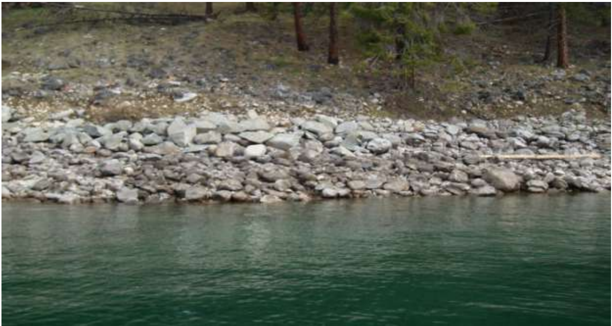
Treatment zone D1 ~ 20 feet single/Double rock
