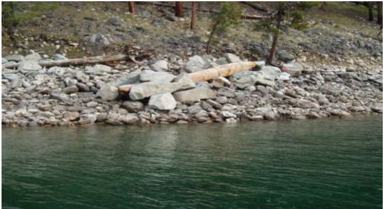
Treatment D3 LWD #1 Place, triple cable and rock (center), LWD #1 Natural back left
