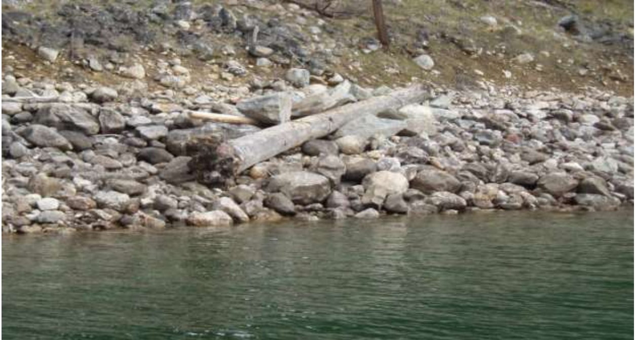
Treatment D3 LWD #2 Placed triple cabled and rocked
