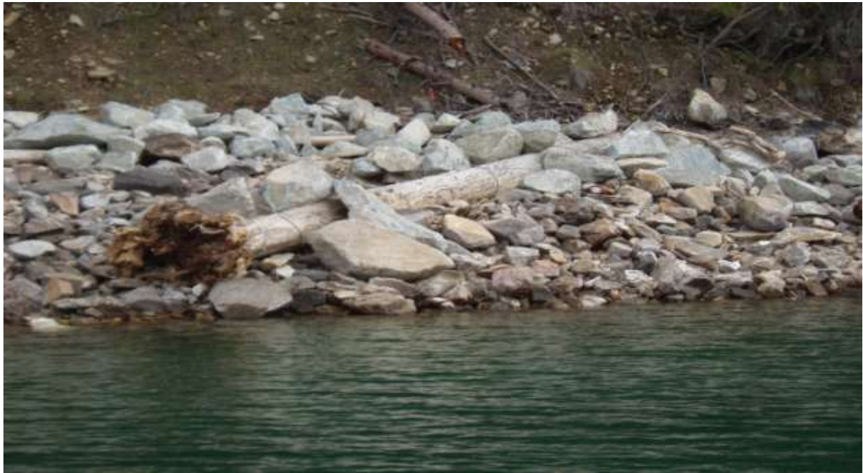
Prince Creek E4 treatment full view of LWD #10 Placed, triple cabled and rocked.
