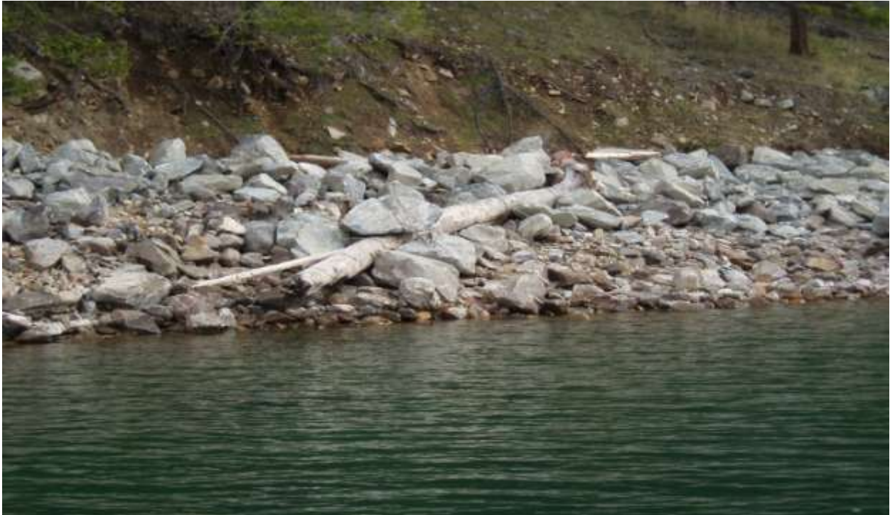
Prince Creek E3 ~30 feet double rock with LWD #8 Placed, triple cable and rockered.
