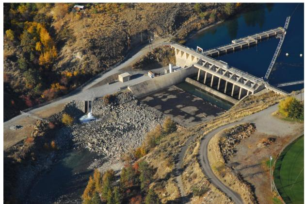
This is a view of Chelan Dam, looking southwest. The Low Level Outlet ends with a concrete outlet structure just downstream of the dam's apron on the right bank (left side of photo). The flow in this photo is 80 cfs.
