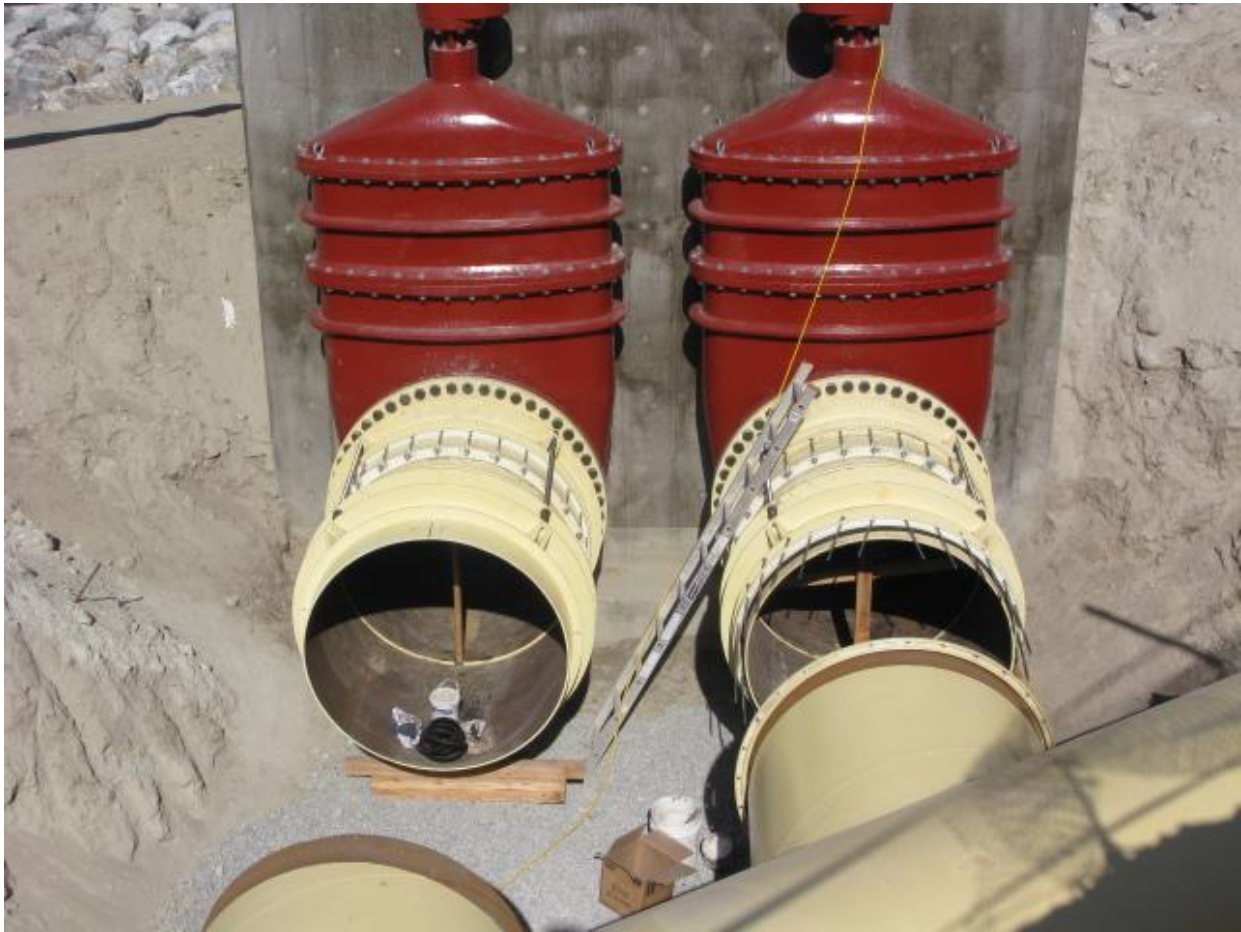
This is a picture of the two 60" gate valves before welding was completed. Picture was taken on May 11 th , 2009.
