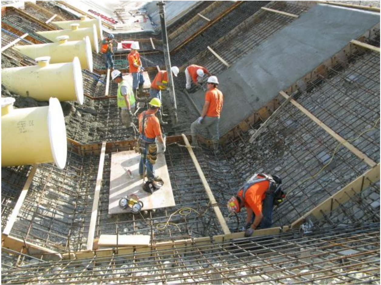
This is a picture of the afterbay at the pump station. This was the first day of 3 days of concrete placements, where 165 cubic yards of concrete was scheduled. Picture was taken on June 1 st , 2009.
