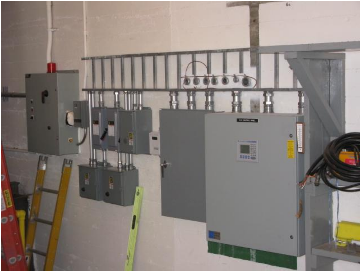
This is a picture of the new panel installation in the valve house at Chelan Dam. Picture was taken on June 4 th , 2009.
