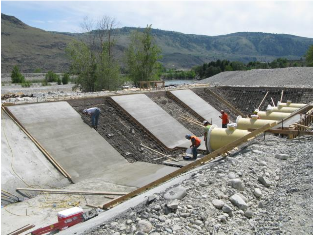
Picture taken of the afterbay at the end of the day, June 1 st , 2009. Notice the contractor's placement method of skipping sections so there would be access to finish the concrete.
