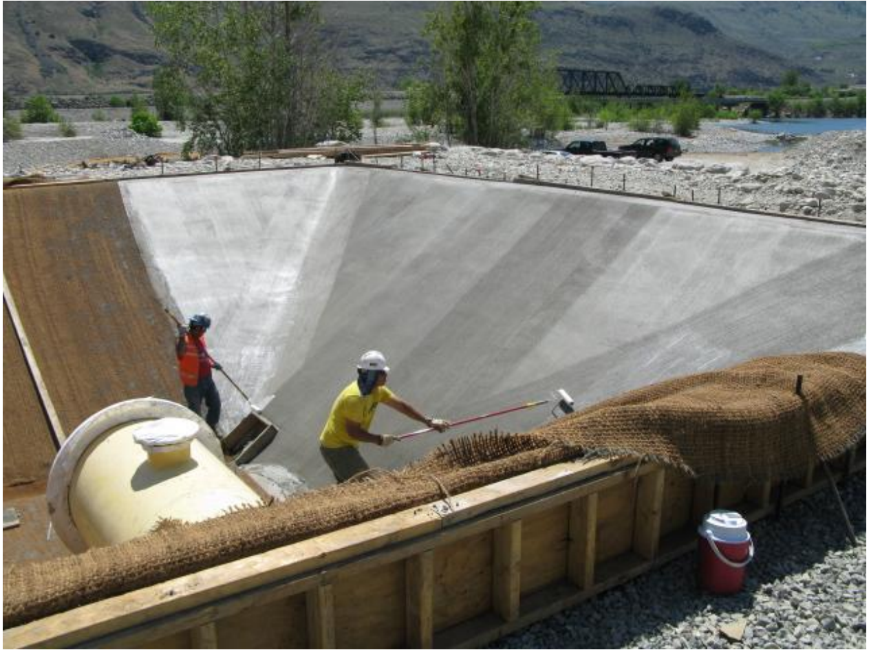
At the end of the day, June 3 rd , 2009, concrete curing was applied to the last concrete placed. Burlap was placed afterward, and kept wet.
