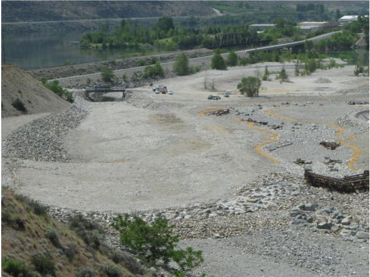
This is a picture of the head end of the spill channel, also taken on June 5 th , 2009. The hydraulic control structure is complete, with its visible grout along the strip at the entrance to the spill channel.
