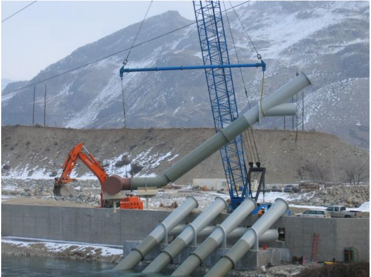
This picture shows the setting of the 5 th pump tube, on 1/27/09.
