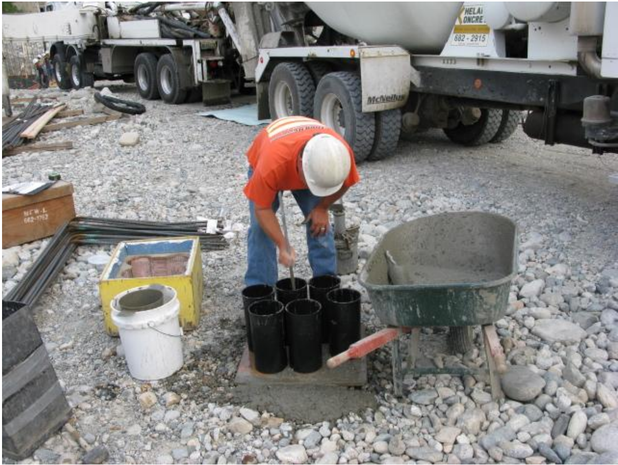
Quality control sampling and testing underway, typical for all concrete placements.
