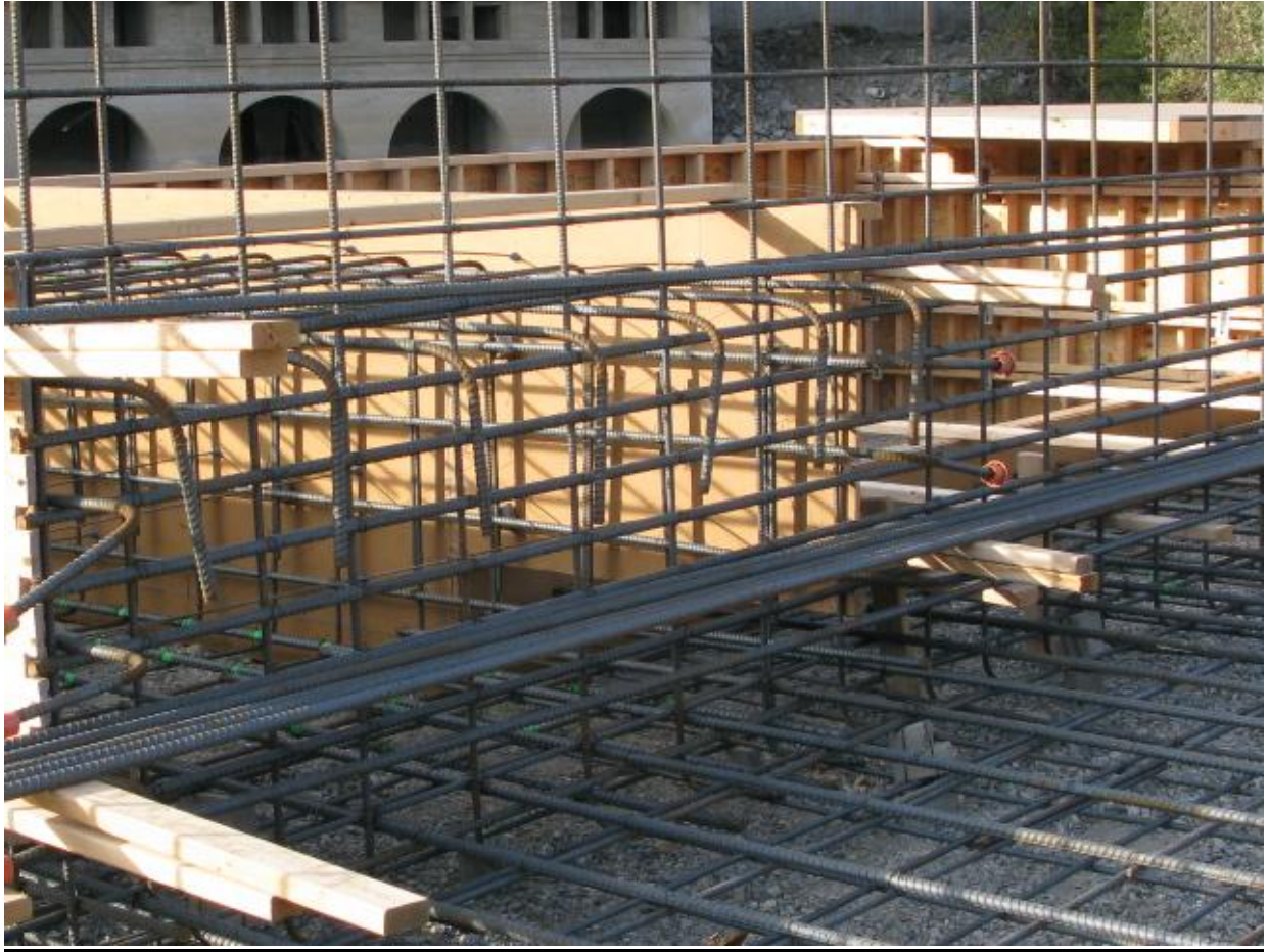
Pump station grade beams under construction. 10/8/08.
