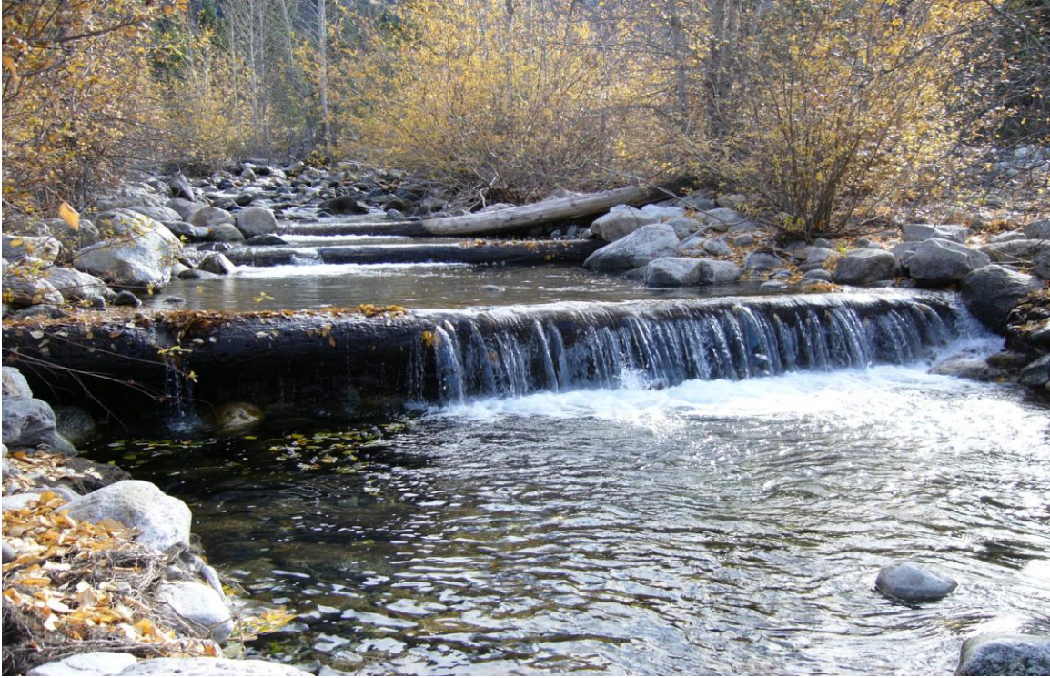
Appendix B. Prince Creek Blockage, (Photos taken in 2007).
