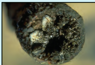
Zebra mussels blocking a pipe
