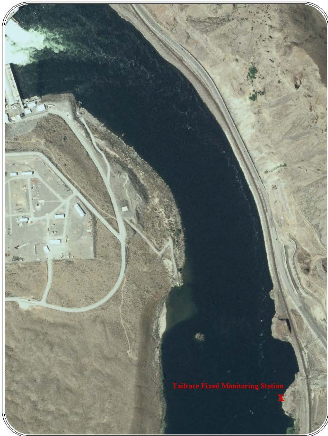
Figure 1-4: Rock Island project, tailrace fixed monitoring station.
