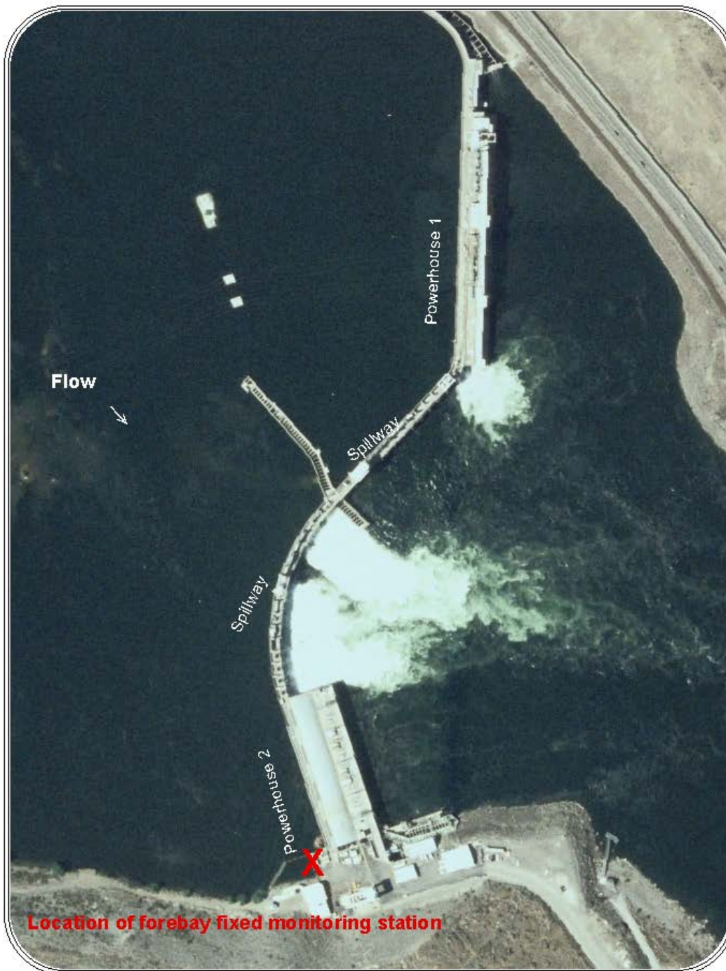
Figure 1-3: Rock Island project, forebay, tailrace and fixed monitoring stations.
