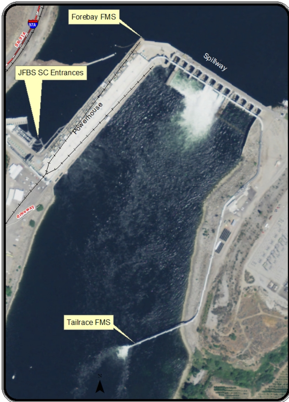
Figure 2. Location of forebay and tailrace FMSs, and JFBS SC entrance.
