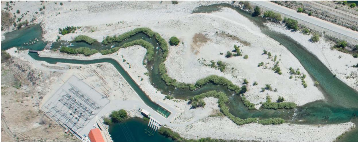
Figure 7-6: Habitat Channel in May 2015.
