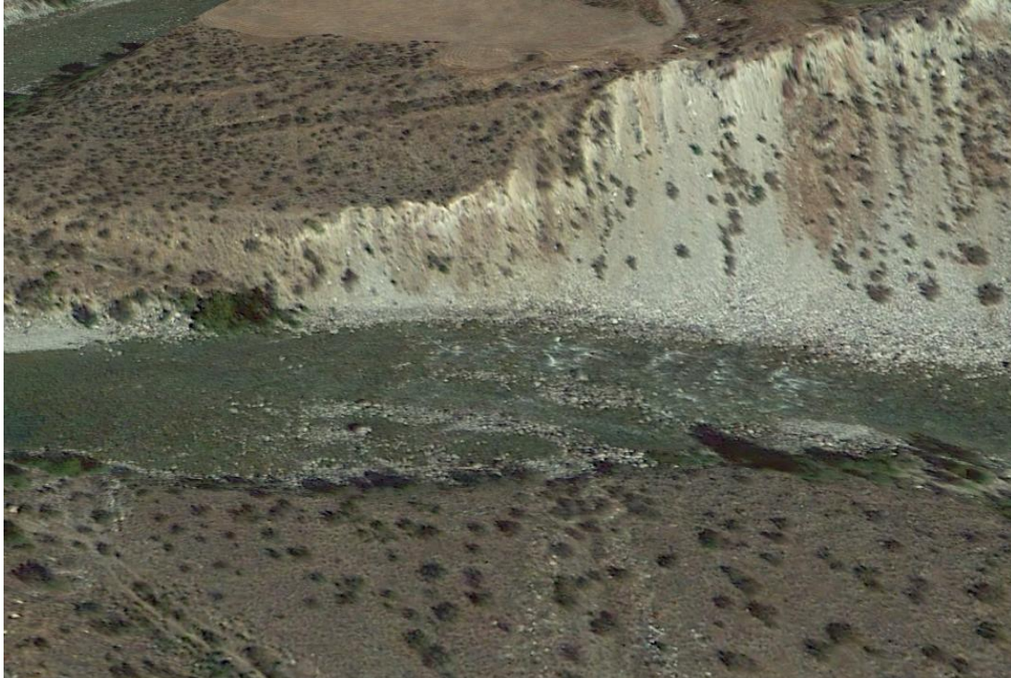
Figure 12. Example of significant obstruction during low flow
