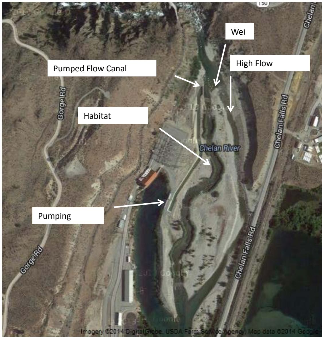
Figure 2. Chelan River Reach 4 showing habitat channel and structures.
