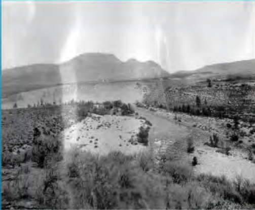
Chelan River before construction, 10/22/25
