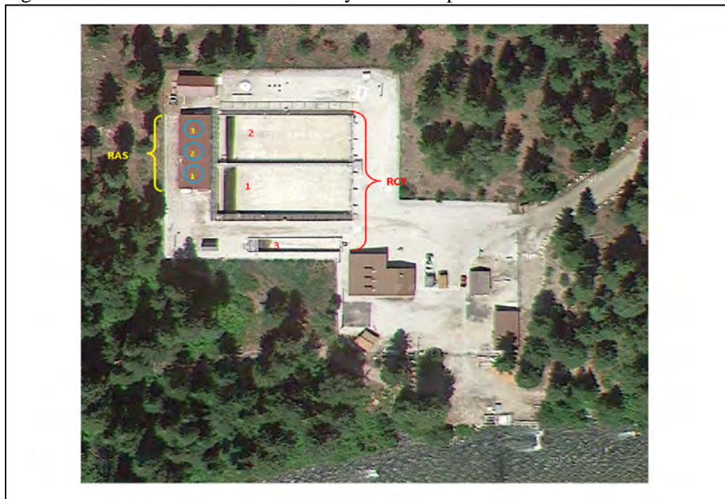
Figure 1. Chiwawa Acclimation Facility site description.
