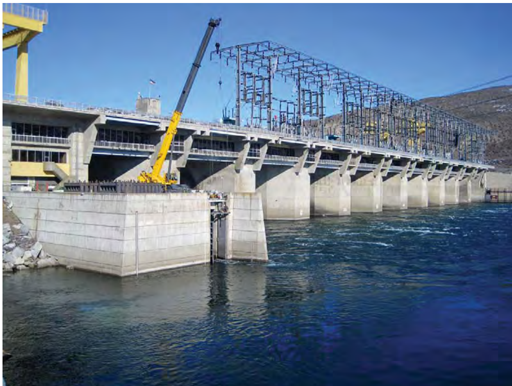
Photo 1: Wells Dam shown with the West fishway entrance in the foreground. (This photo was taken by Jacobs Engineering during the trolley testing in Feb 2011)
