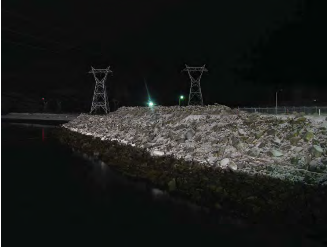
Photo 7: This photo shows the low tailwater condition used for Tests 1 and 2, roughly El. 706.5'. (Photo by NHC)
