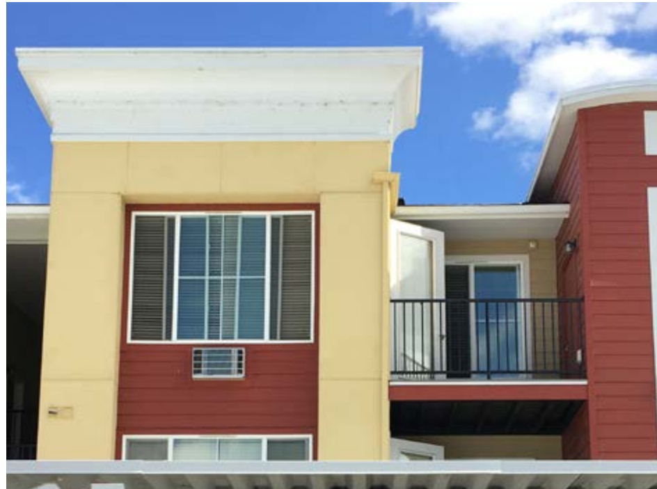
Doors and windows open on a chilly day may point to unauthorized cryptocurrency machines that need cooling.
