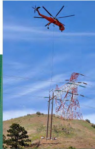
Specialized "flying crane" helicopter ferries in one of the structures for the 5.8-mile Entiat Transmission line constructed in 2012.
