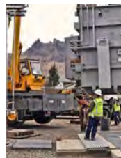
About the back cover: A new transformer goes into place at Okanogan Avenue Substation in Wenatchee.
