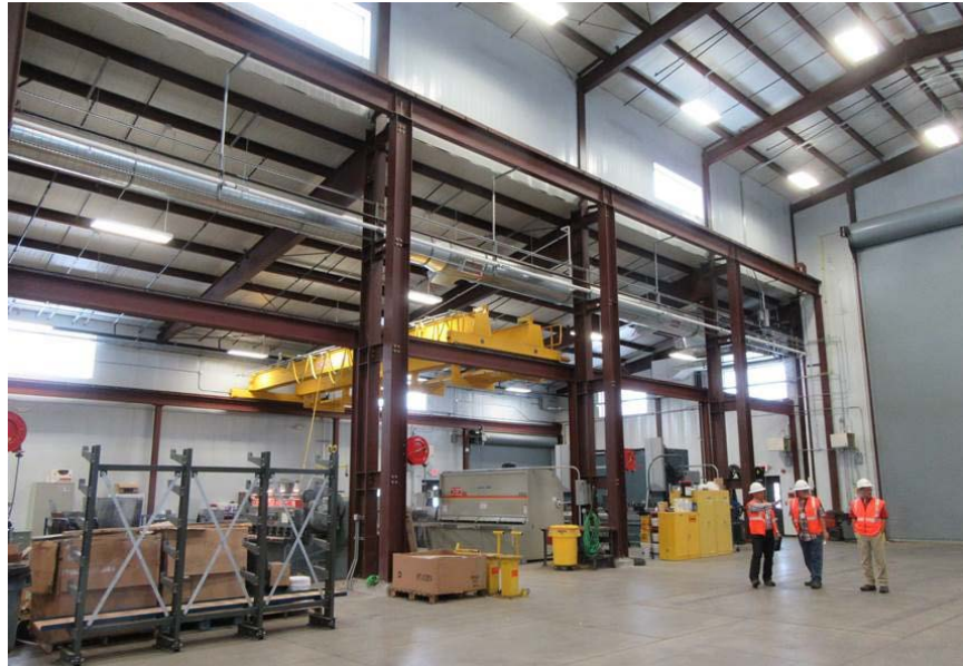
Grant County PUD – Wanapum Fab Shop
